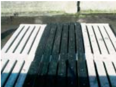
Rubber strips secured to concrete
