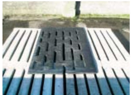
Perforated rubber mats over the slatted area
